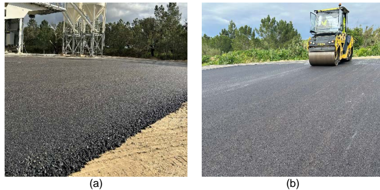
Fig. 1– Mixtures applied in the full-scale pavement trial: (a) AC20 mixture, (b) AC14 mixture.
